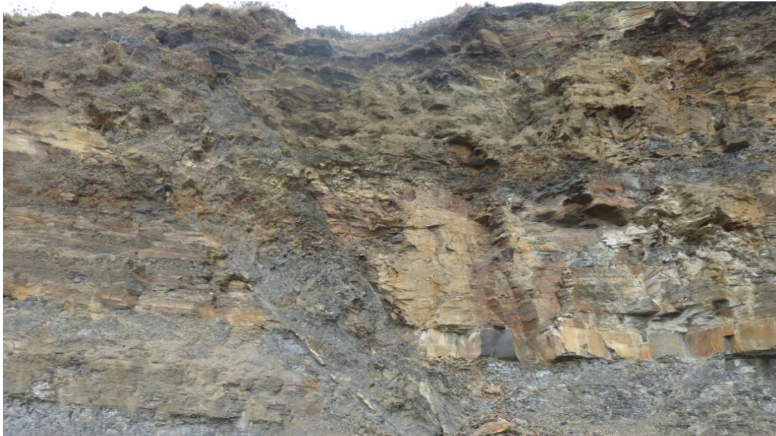
A fault zone is clearly visible in this cliff face
