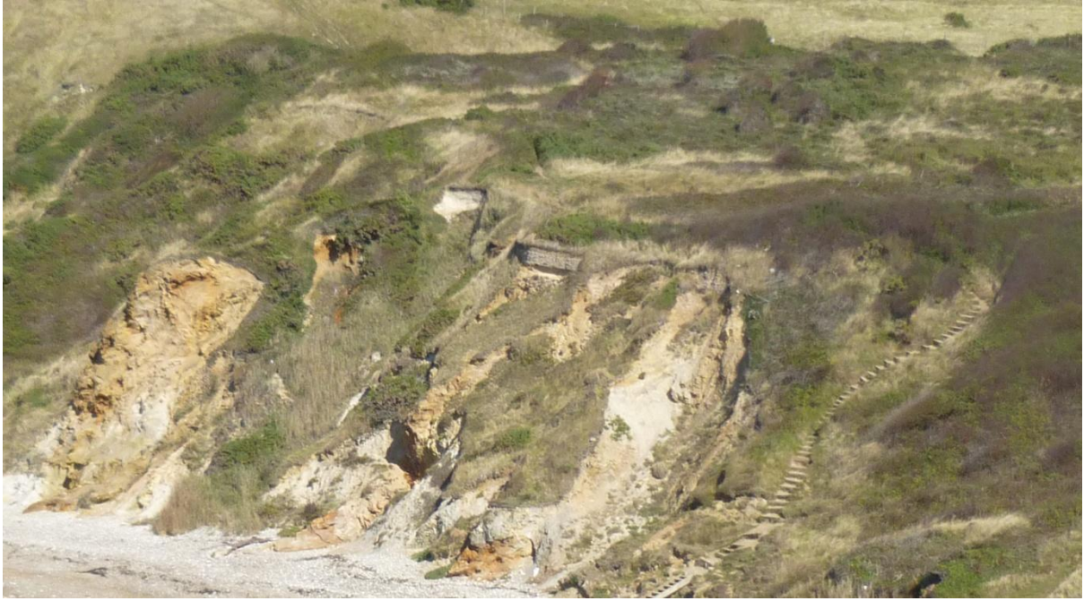
Wealden beds with landslip caused by overlying Gault lubricity
