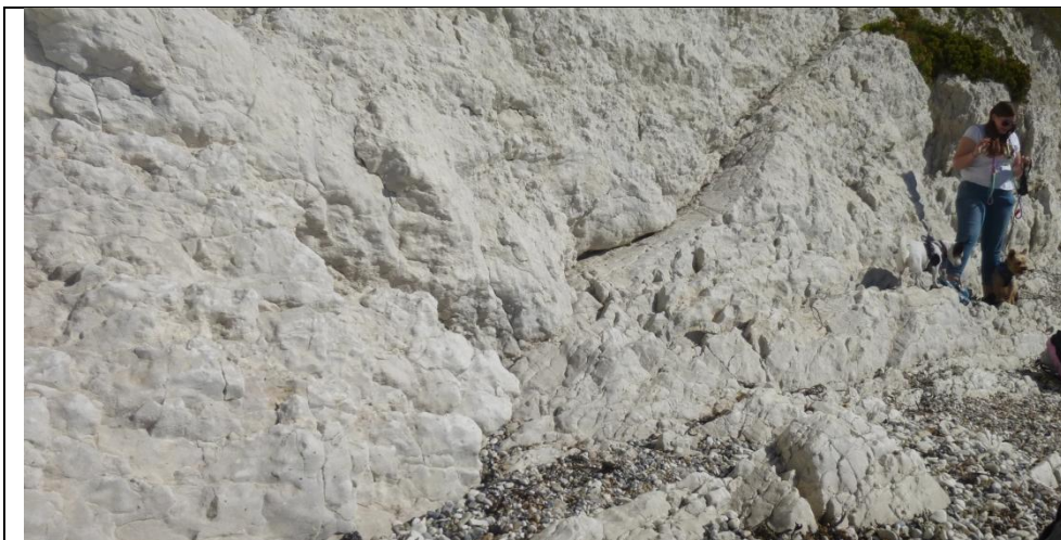
This cliff face is a major fault. Slickensides are very visible
