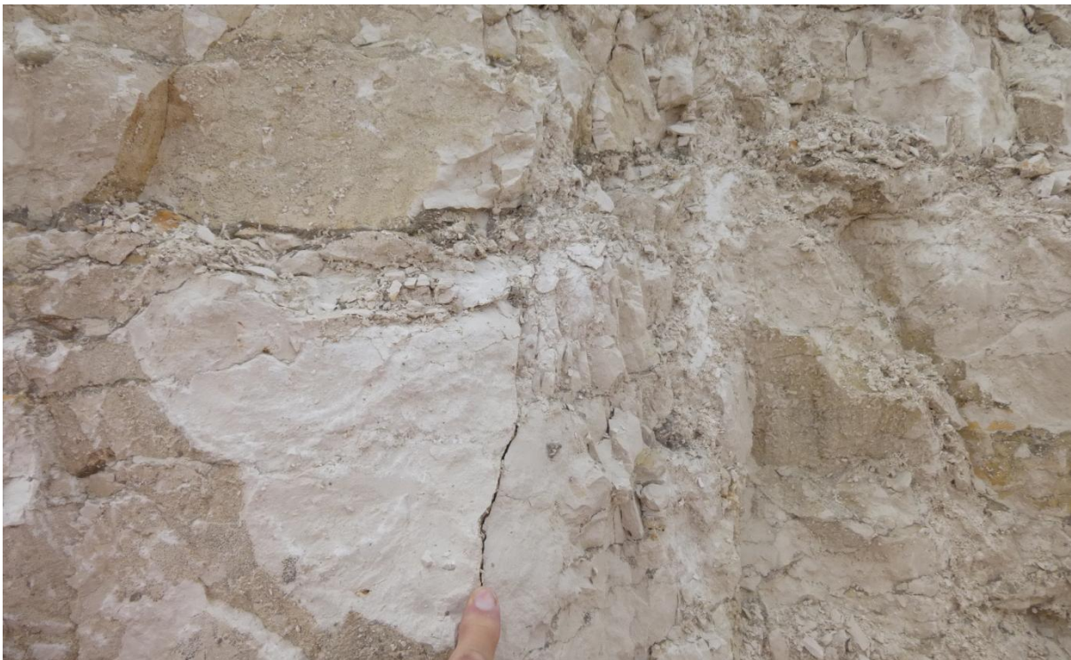
cm displacement fracture
