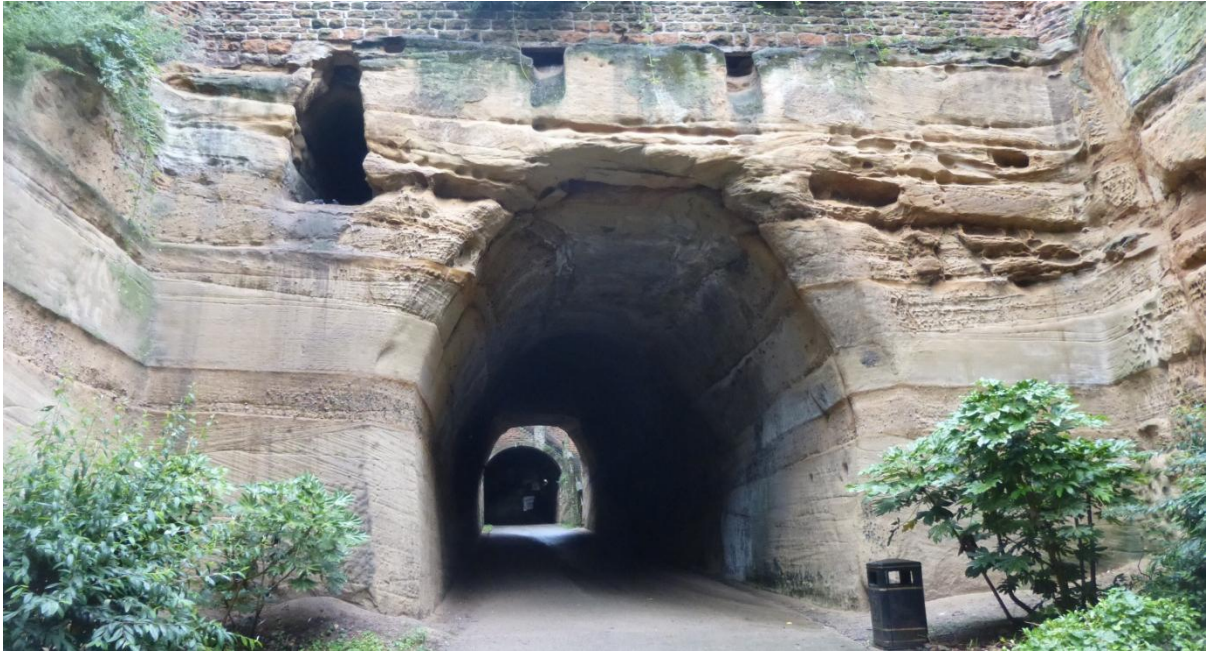
View of the tunnel from the south end
